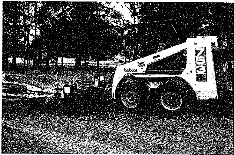
FIGURE 2. The "Harley Rake" on this skid-steer loader is mixing soil amendments with native soil.
